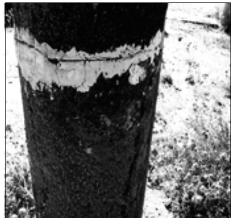
Figure 3: The use of Portland cement to restore limestone and basalt columns at Abila.
