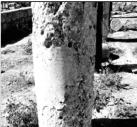
Figure 3: The use of Portland cement to restore limestone and basalt columns at Abila.
