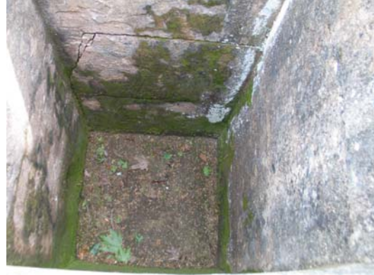
Fig. 6: The interior of the tank
