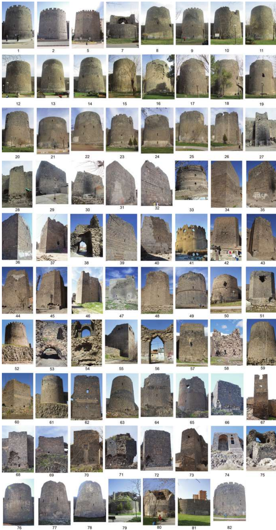
Figure 6. View of the exterior surface of the bastions.
