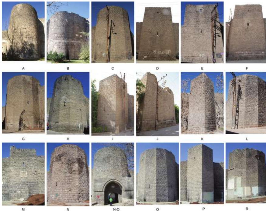
Figure 7. View of the exterior surface of the bastions.
