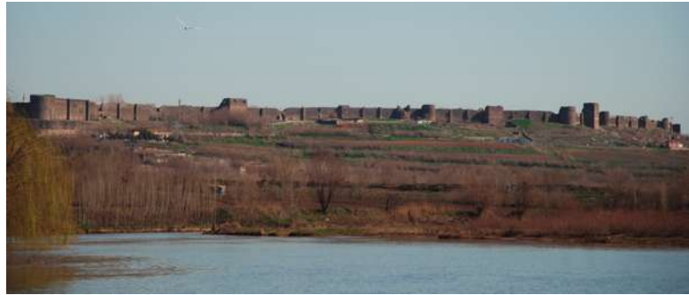
Figure 3. A view of southeast part of Diyarbakir City Walls
