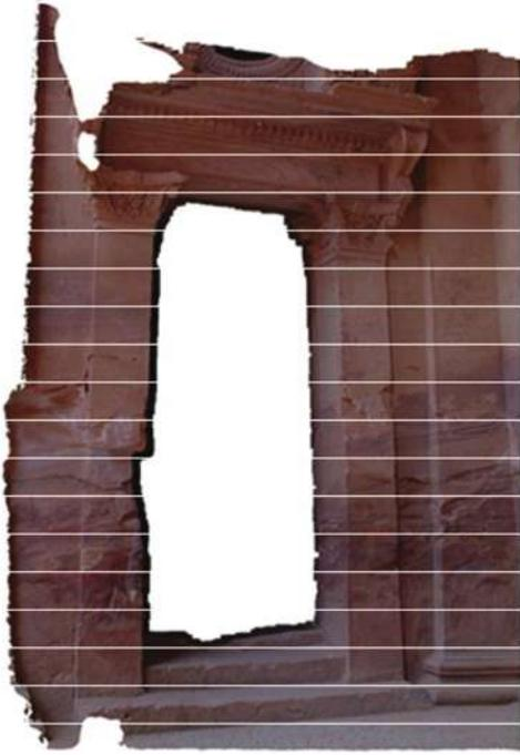
Figure 13. True orthophoto of the right door of Alkhsneh with two millimetre object size resolution.
