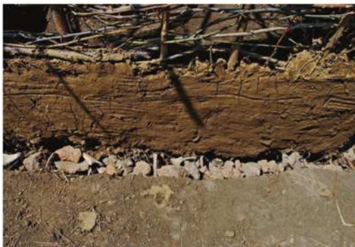
Figure 17: Detail with the daubing of the north-eastern wall. Sultana-Malu Roşu experiment.
