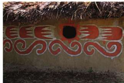
Figure 25: View of the north-eastern side of the experimental building from Sultana-Malu Roșu.
