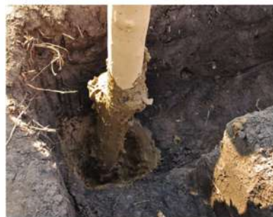
Figure 10: The north corner post (without bark and plastered with clay). Sultana-Malu Roşu experiment.
