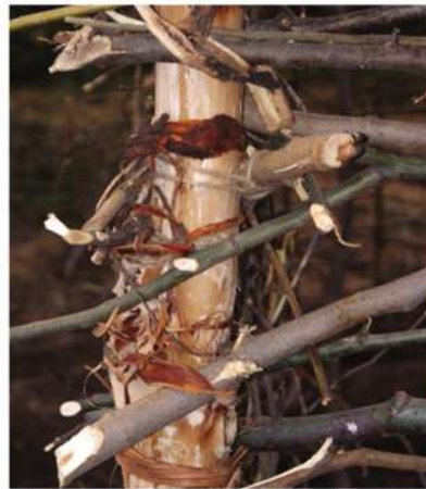
Figure 14: Detail of the wall structure fixed with willow bark. Sultana-Malu Roșu experiment.
