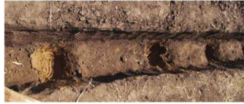
Figure 9: The north-eastern foundation trench and post holes. Sultana-Malu Roşu experiment.
