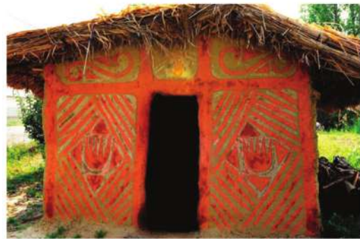
Figure 24: View of the north-western side of the experimental building from Sultana-Malu Roșu.
