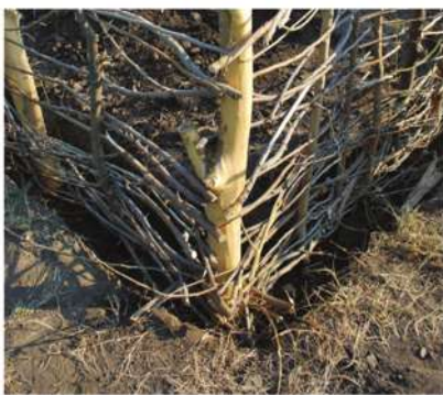
Figure 13: The south-western corner and wall structure sited in the foundation trenches. Sultana-Malu Roșu experiment.
