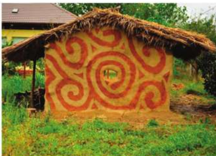
Figure 23: View of the south-eastern side of the experimental building from Sultana-Malu Roșu.
