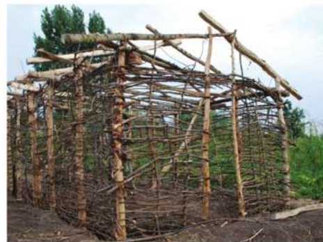
Figure 12: The wooden structure of the experimental building from Sultana-Malu Roşu (North view).
