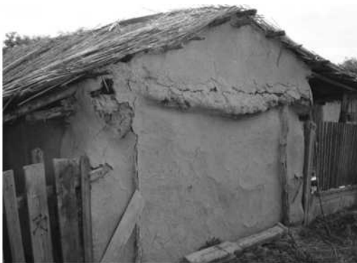
Figure 7: Traditional construction made of wattle and daub from Sultana village.
