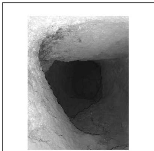
**Figure 6: A spirally stepped-down shaft on north flank of the creek valley Location No. 5.**
