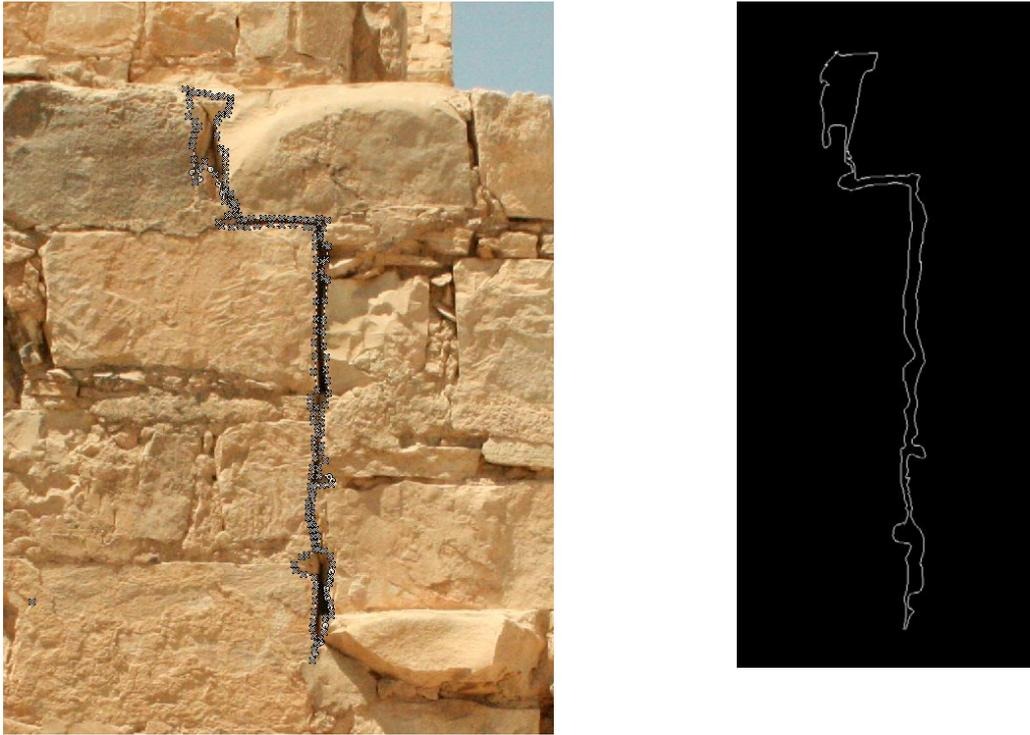
Figure 6. Quantification and 3D modeling of the cracks at the studied wall in Amra palace using photogrammetry approach.
