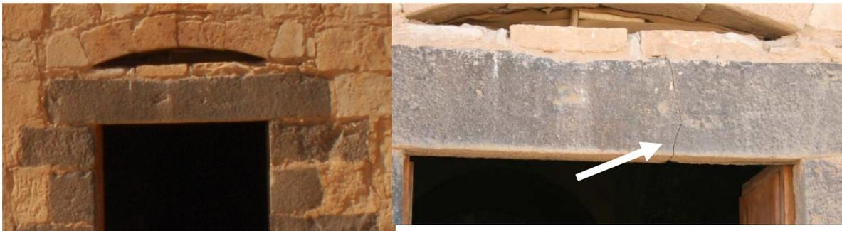
Figure 2. Images for the main entrance door of Amra palace taken in different epochs the white arrow in right photo shows a serious crack was created in the upper part of the door.
