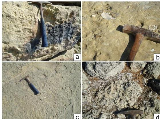
Figure 7 Detailed view of the blocks employed in the roman pier: a) compact whitish-yellowish biomicrite (southern curtain); b) slightly glauconitic whitish-greenish biomicrite with sparse pectinids (southern curtain); c) greenish biomicrite with fossils and horizontal tubular bioturbations (inner concrete); d) biodetritic limestone rich in gastropods and bivalves (inner concrete).
