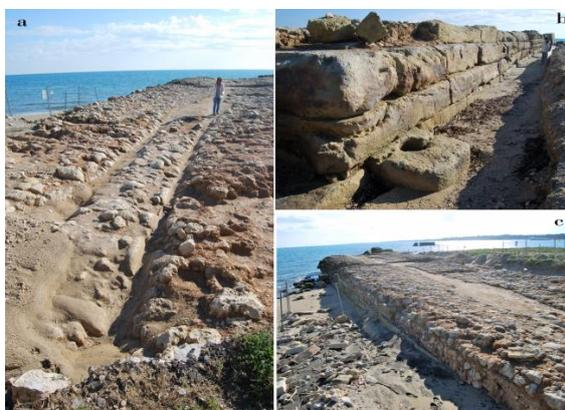
**Figure 4** Some images of the ancient monument showing: a - the inner concrete, b - the southern curtain made by Pietra Leccese blocks and the mooring ring projecting from the inside face of the pier; c - the northern curtain.
