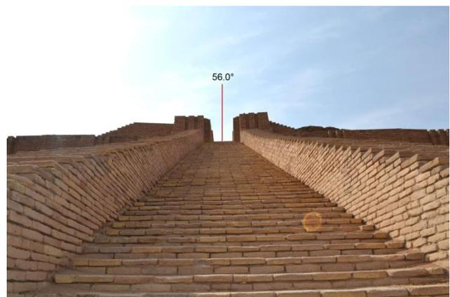
Figura 5: Measurement of the frontal staircase of the Ziggurat (photo by the authors).
