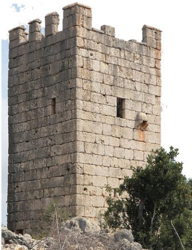
Akkum Tower; front and side facades
