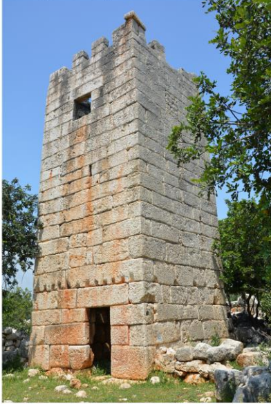
Gömeç Tower; front and side facades
