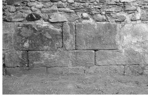
Figure 5. The Hellenistic wall in Hypaipa
