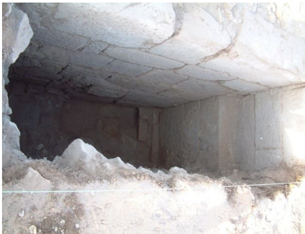
Figure 8: Wall in the proposed bath with details of construction and possible mud brick floor
