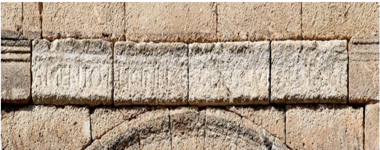
Figure 3. Limestone Details in Arch of Berà
