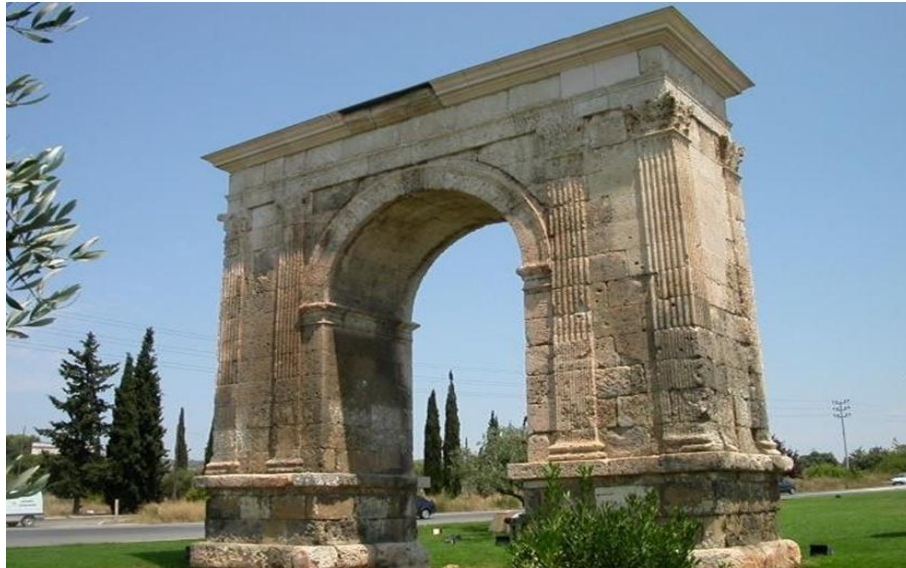
Figure 4. The Current State of Arch De Bera
