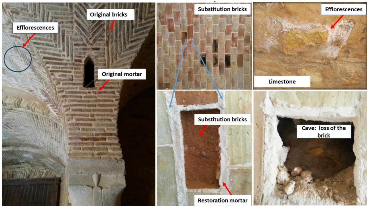
Figure 2. Building Materials and Decay Patterns
