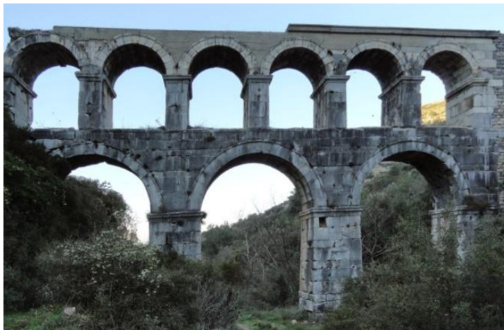
Figure 3. Pollio Aqueduct Bridge, Aydin
