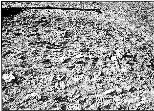
Figure 5. Pavement in Trench 2.
