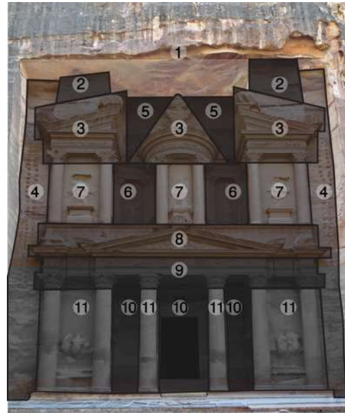
Figure 13. Photographic illustration showing the probable different sequenced stages (1-11) for the cutting order and final decoration finishing of el-Khazneh two floors' façade.
