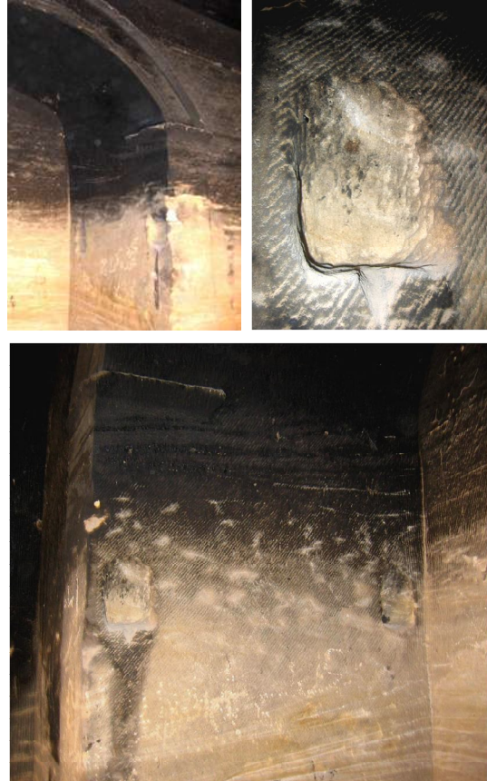
Figure 9. Similar cut slots to el-Khazneh from the second tomb level at the back wall of the inner space at the Obelisk tomb.
