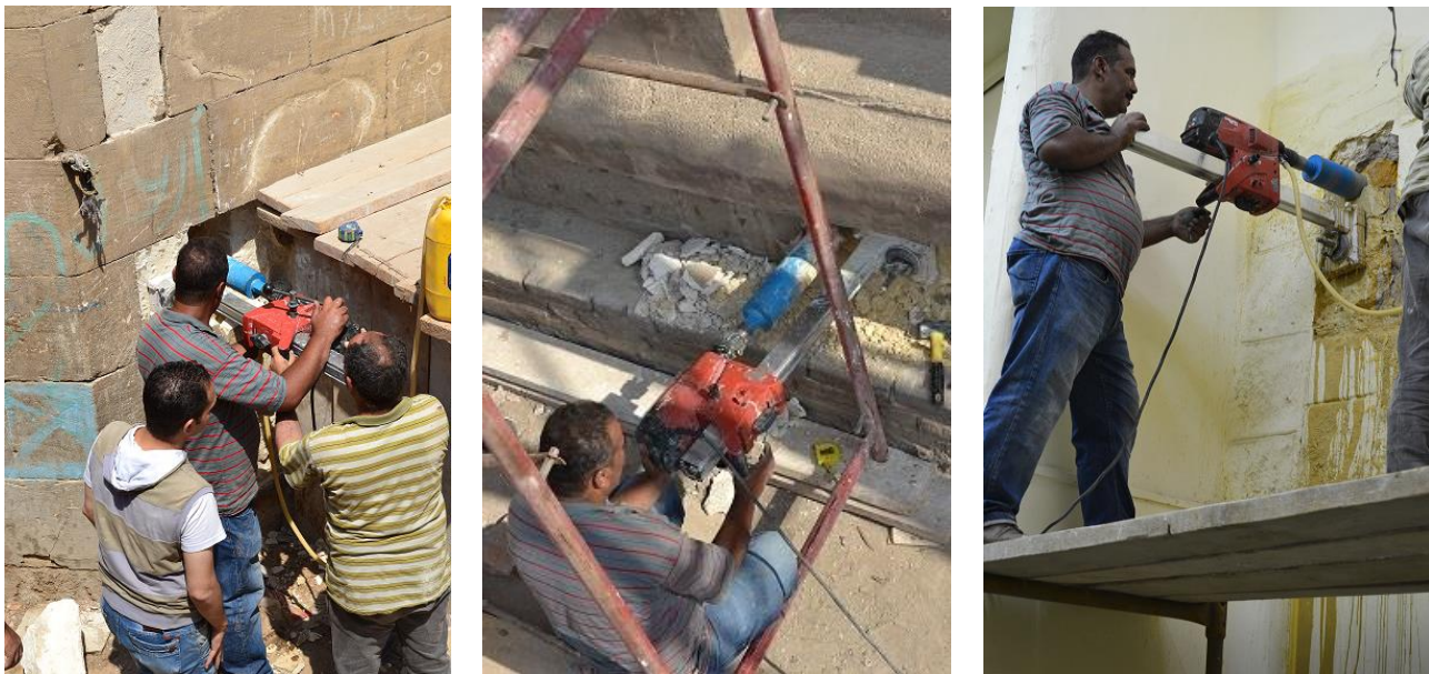
Figure 5. Extracting of the investigated core samples
