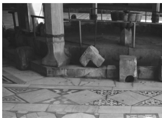
Fig. 11: The slabs which are around the fountain and always exposing to the water do not suffer from any deformations produced by expansion.
