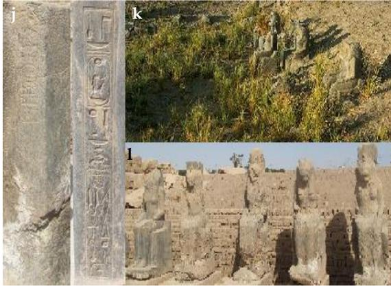
**Figure 3** details of deterioration at the diorite statues at Mut temple.
