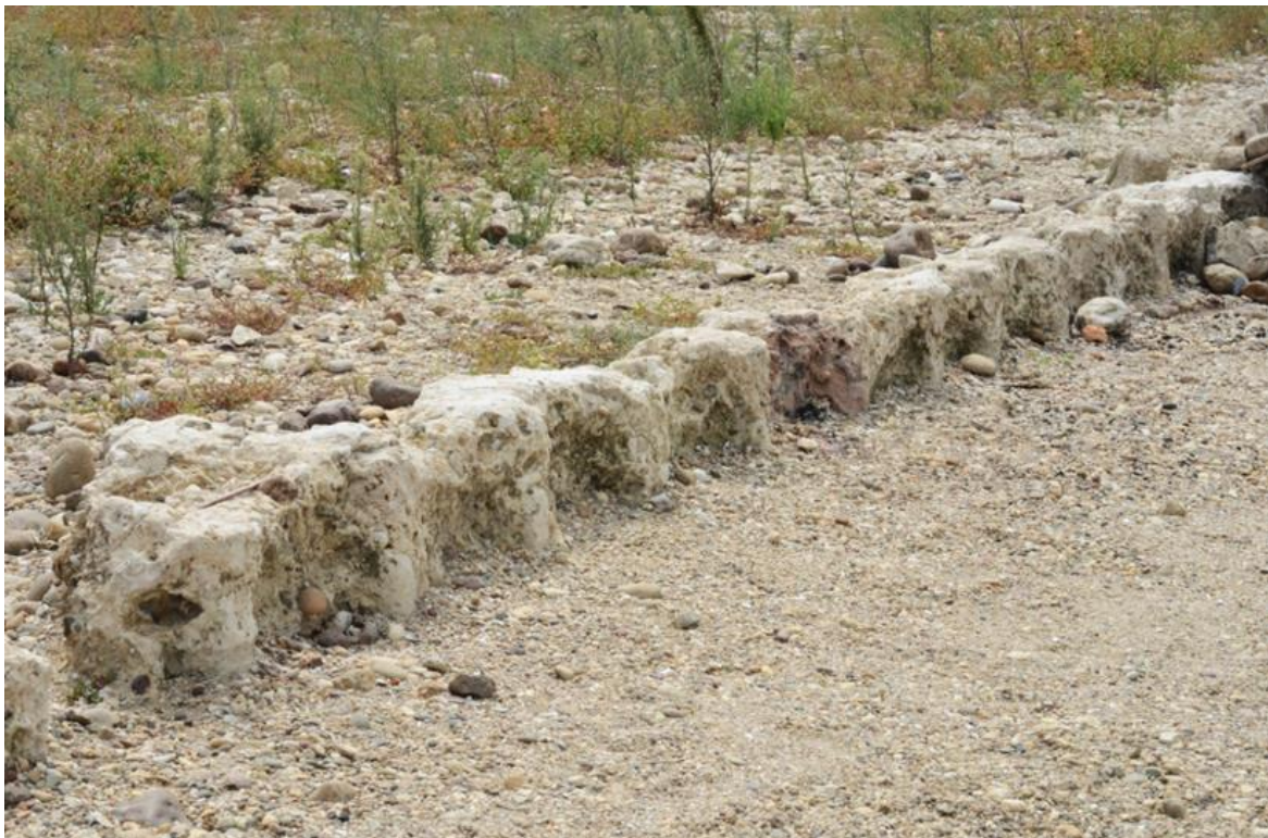
Figure 4d. A close up view of the embankment.
