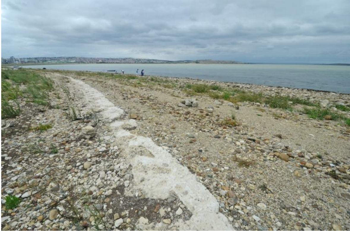
Figure 4a. Embankment made of pebbles, sand, sand stones and limestone.
