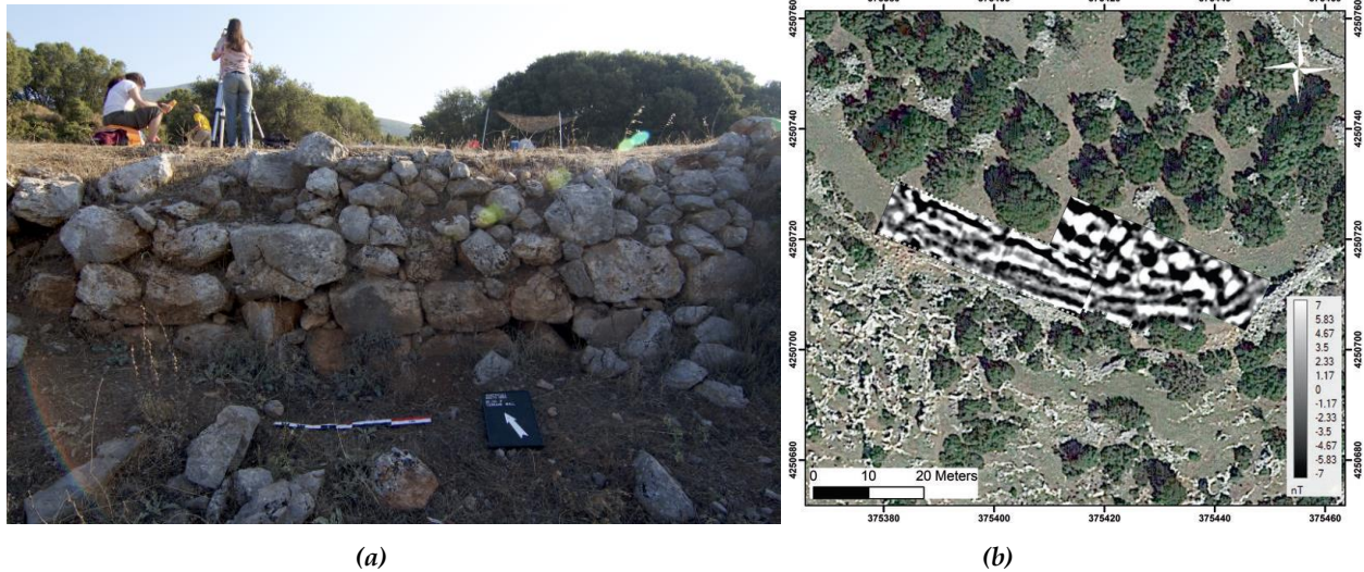
Figure 19. (a) Site-wide retaining wall at Southern Terrace, (b) Magnetic gradient at Southern Terrace (a. Photo by I. Roy, b. Image by G. Tsokas in Levy et al. , 2018)
