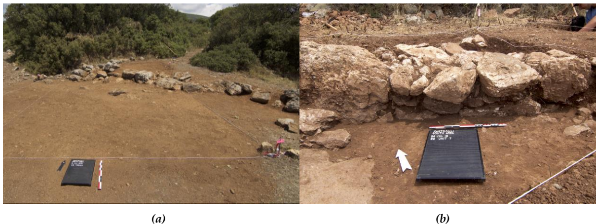
Figure 22. (a) Building 2 West with Wall A1 Unit 1, (b) Building 2 East with Wall B2 Unit 5 (Photos by A. Krohn)
