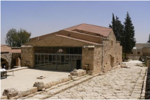
Figure 1. General view of the Virgin church and the Hippolytus Hall with new shelter
