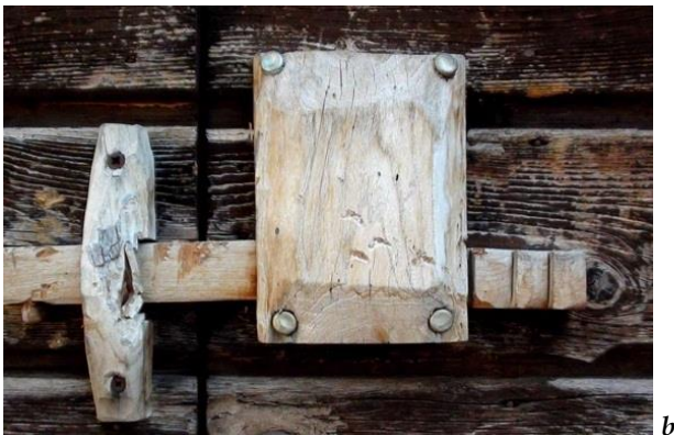
Figure 7 a) Wooden lock from Karpathos (Dawkins, BSA, X, 1902-3, 192-3, fig.8). b) Hand-crafted wooden door lock from the traditional village San Benedetto in Perillis, Italy (Soldati, 2012, https://www.youtube.com/watch?v=9zp2Xi5OnUM ).
