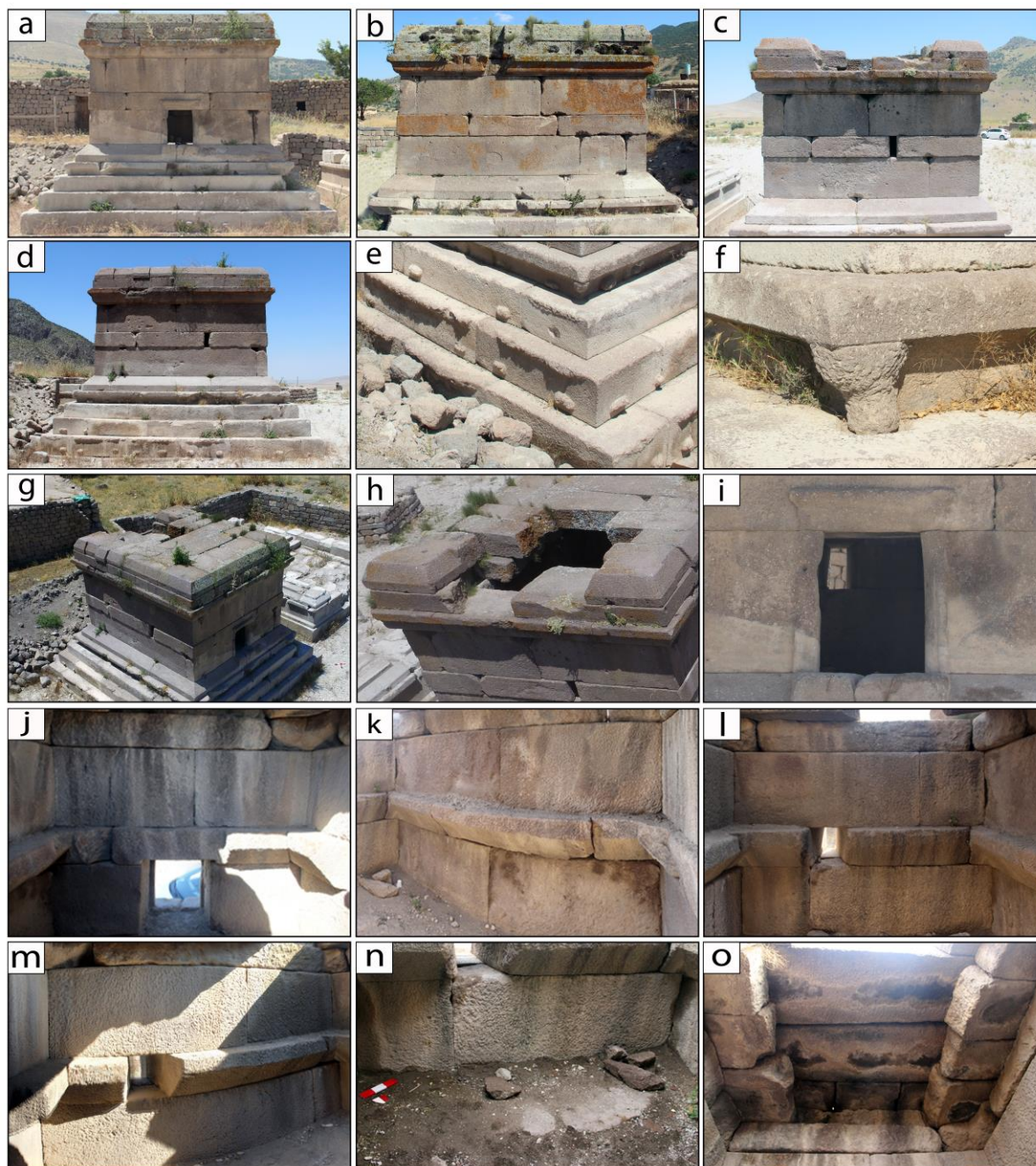
Figure 3. Facade and interior views and details of the mausoleum; a) northeast facade, b) northwest facade, c) southwest facade, d) southeast facade, e) projections called tenon, f) stylized plant figures, g) top cover, h) pedestals found at the corners of the southwest facade and missing top cover stones, i) entrance gate of the tomb, j) northeast wall, k) northwest wall, l) southwest wall, m) southeast wall, n) earth-filled ground, o) stone consoles and ceiling.
