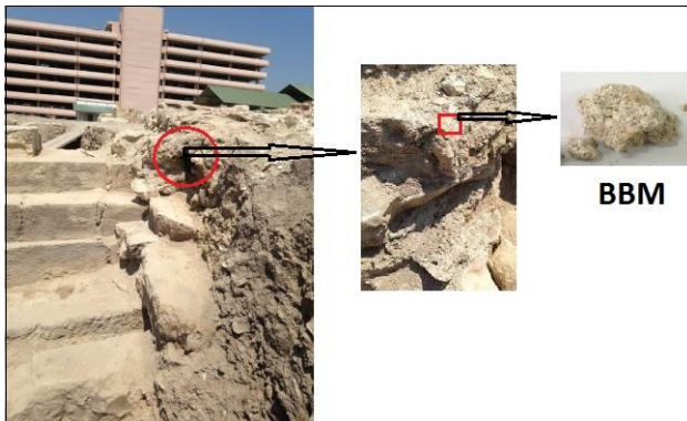
Figure 3. Bouleuterion blockade mortar between stones (BBM).
