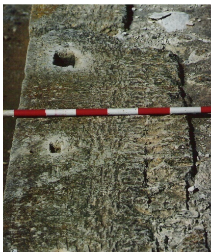
Fig.13-14. Ashlars from Kition showing small mortises at the top of the orthostats
