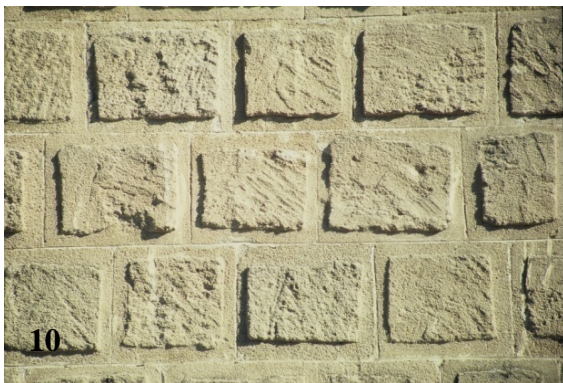
Fig.9-10: Drafted margins in Late Bronze Age masonry (1200 BC – Fig.9) and in a colonial building (19th century AC – Fig.10)
