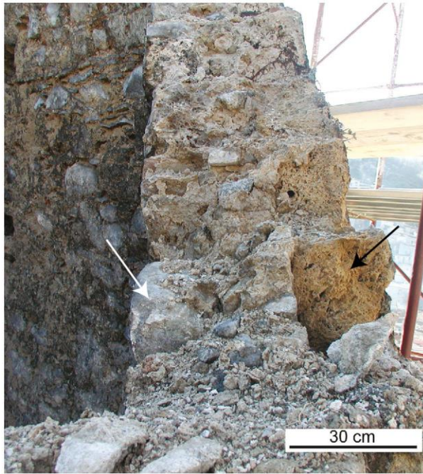
Figure 3. View of the broken original masonry. Note the wall lot typology of the structure in which the external layer is made up of blocks of local calcareous tufa (black arrow), and the internal layer of riverine blocks (white arrow).
