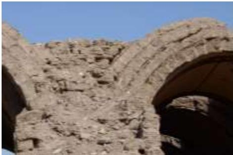
Figure 3. The adobe vault of the storeroom of the Ramesseum temple composed by four courses, the filling between the adjacent vaults can also be noticed.
