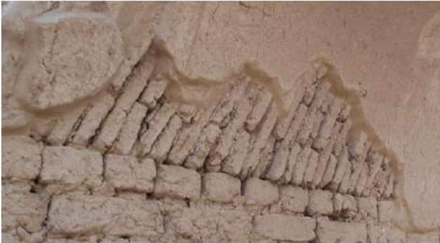
Figure 2. Mud-bricks laid tilted in an Ancient Egyptian barrel vault (in the storerooms of the Ramesseum temple).
