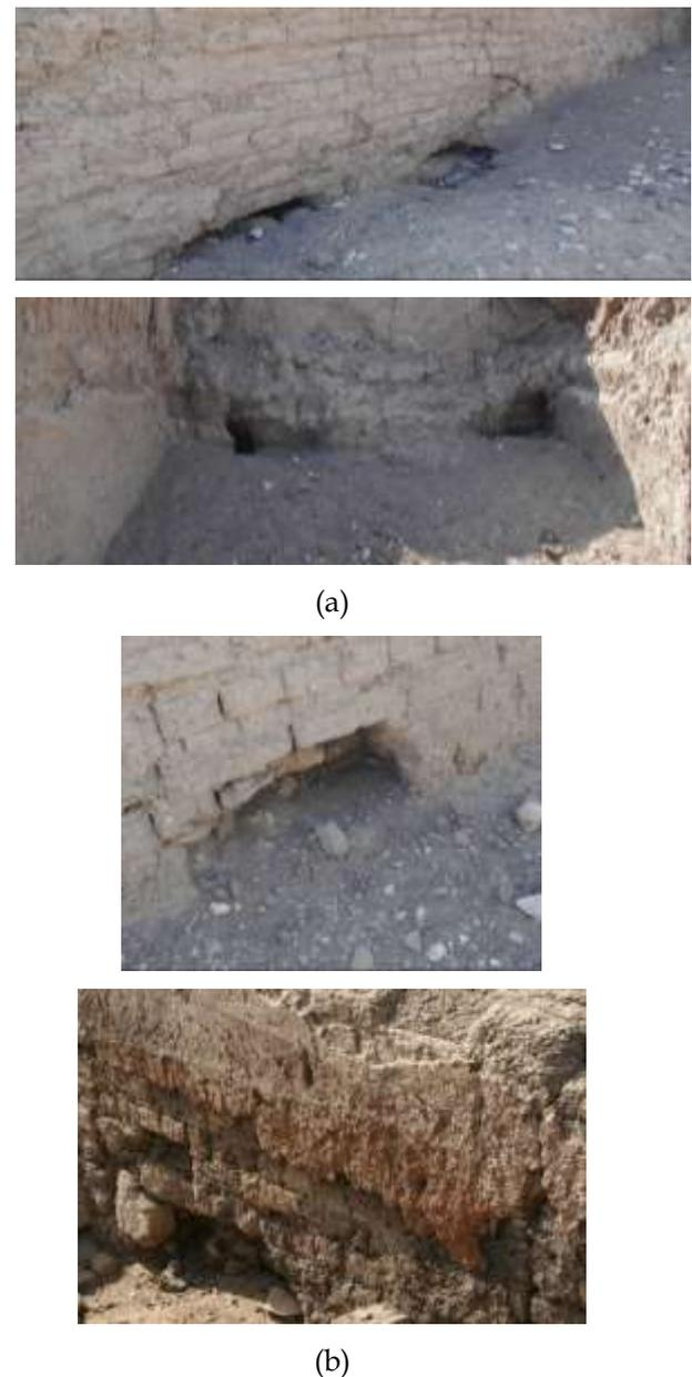
Figure 16. Holes made by animals (a) Sety I storerooms and (b) the Ramesseum storerooms.
