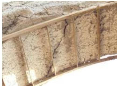
Figure 30. Large cracks at places of strengthening intervention.
