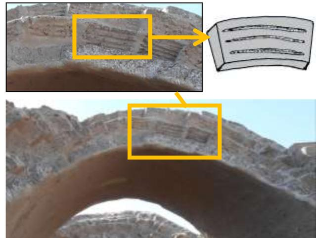
Figure 5. Bricks made with grooves to ensure the brick-mortar bond. The storerooms of the Ramesseum temple.
