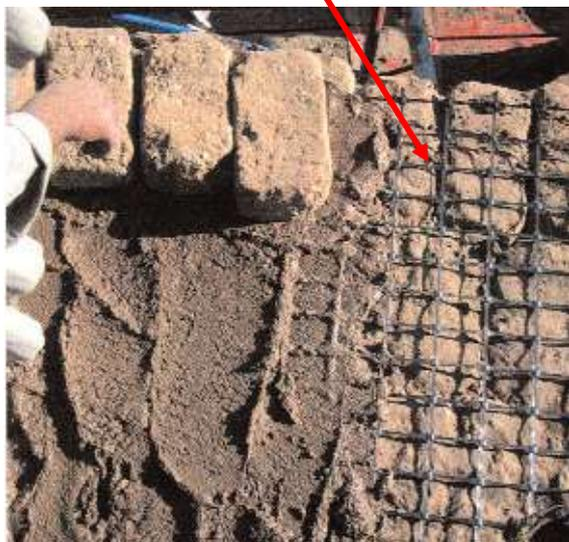
Figure 32. The application of polymer grids between adobe wall courses in Shunt el-Zebib in Abydos.
