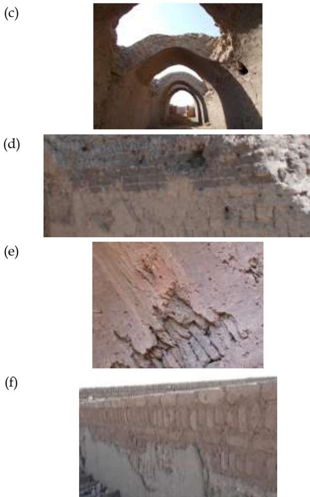
Figure 15. Many symptoms of damage in the storerooms of Sety I and the Ramesseum temples (a) cracking, (b) partial collapses, (c) holes widening, (d) erosion, (e) plaster detachment and (f) restoration using incompatible materials.
