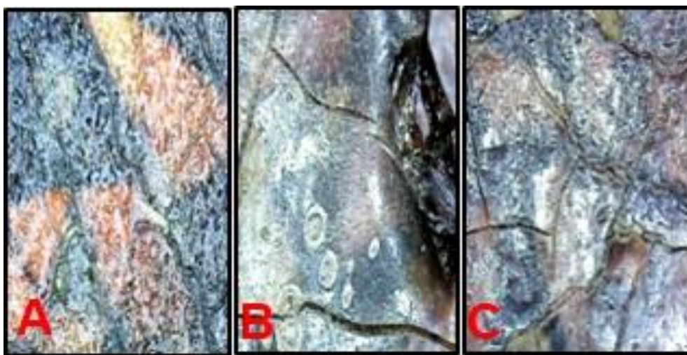
Figure 8 Portable digital USB microscopic examination, showing deterioration of varnish layer: (A) Discoloration (B) Congregation of varnish and cracks (C) Micro cracks, 1000X.
