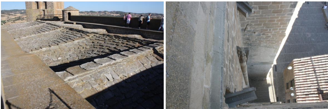
Figure 6. S. Saturnino de Artajona. Roof, downspouts and gargoyles.
