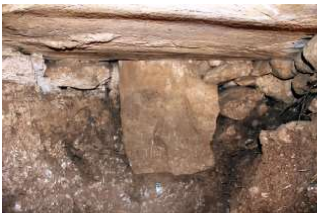
Figure 12. Tomb A: the southern extension with its monumental roofing slab and another large rectangular slab in its southern wall. Photo A. Sideris.
