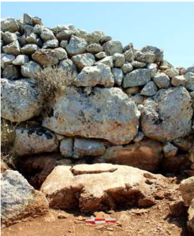
Figure 28. The W-NW section of the fortification wall erected upon the bedrock. It shows, at least, two phases of construction. Photo A. Sideris
