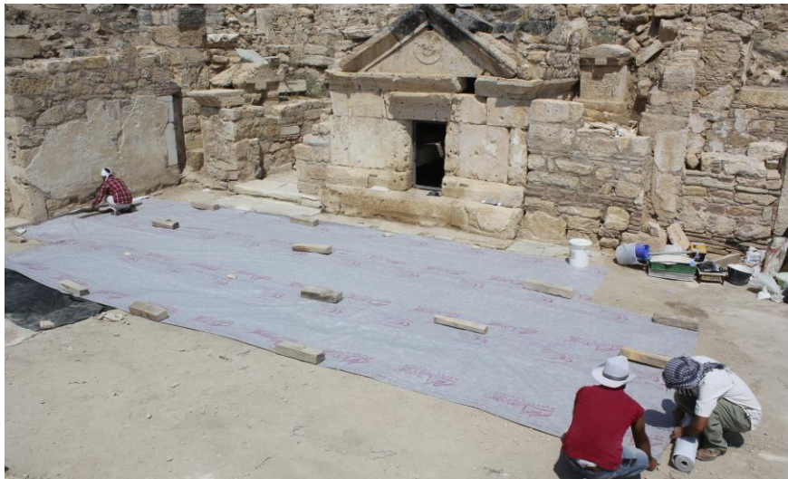
Figure 19. Panels were covered with Gore-Tex geotextile.
