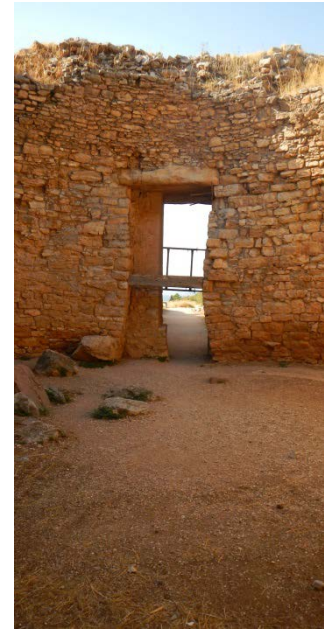
View of Stomion from Interior (note Relieving Triangle)
