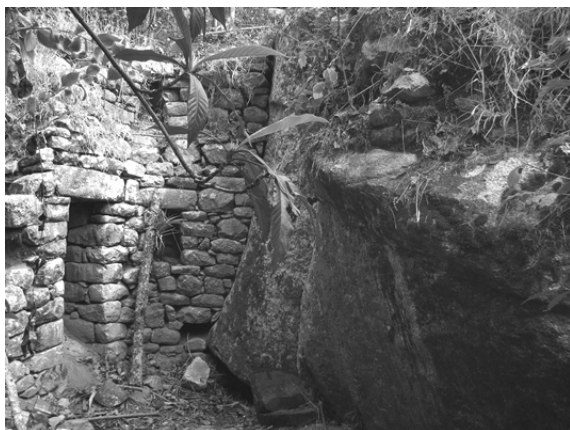
Figure 7 A curved masonry wall with a door, niche and window adjoins an in situ boulder in the River Intihuatana tower. The cave entrance is to the right of the stone.
