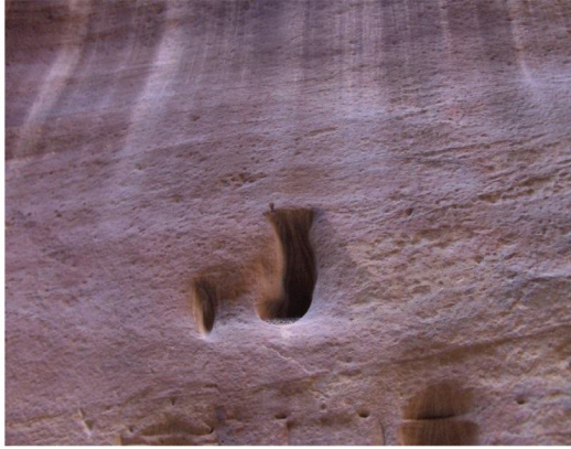
Figure 2. The "Luck Niche" in Siq area, tour guides and tourists keep throwing stones, which caused more erosion of the sandstone
