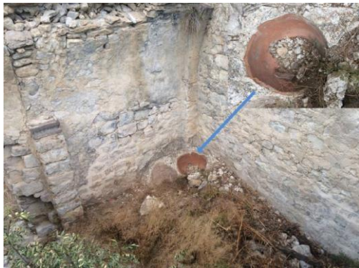
Figure 20. In the Frescoed Chapel, wine cubes (structure A).
