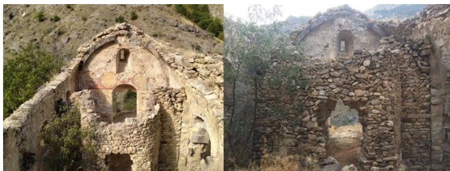
Figure 8. The Frescoed Chapel's north view and interior detail (structure A).
