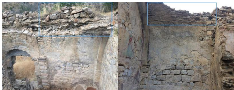
Figure 6. Remains of structure A's vaulted roof and view of wall structure.
