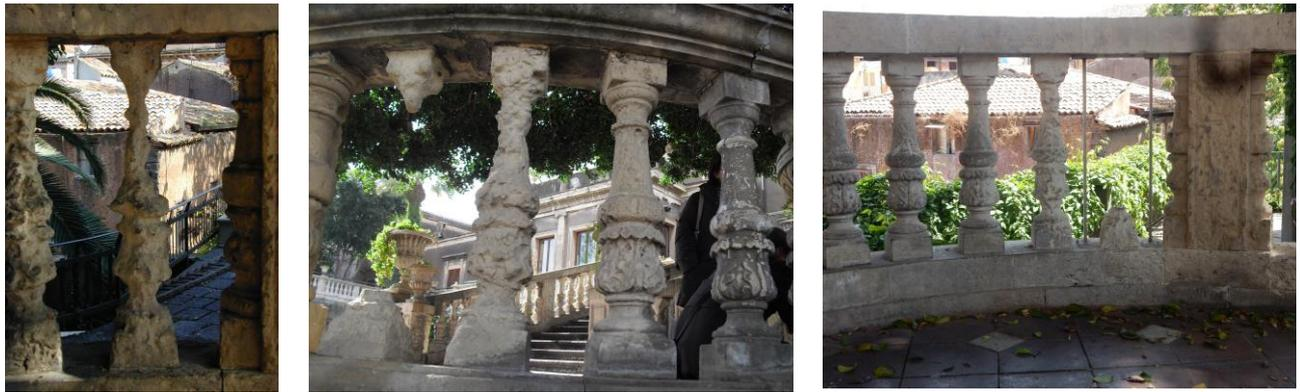
Figure 13. Three stages of decay: on the left photo of 2001; in the centre, the baluster without spindle (February 2015) and on the right, a minimal intervention was chosen, inserting sheets of stainless steel supporting the handrail.
