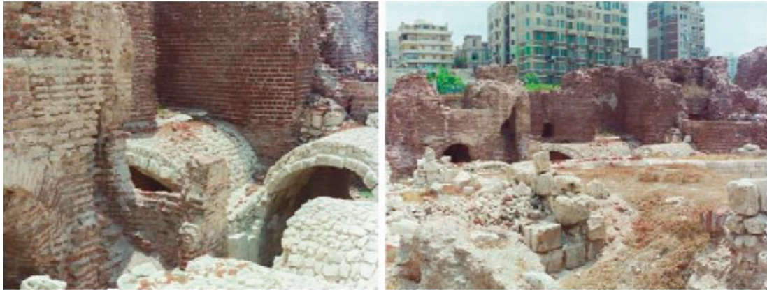
Figure.2. The structural damage of the remains and masonries is obvious.
